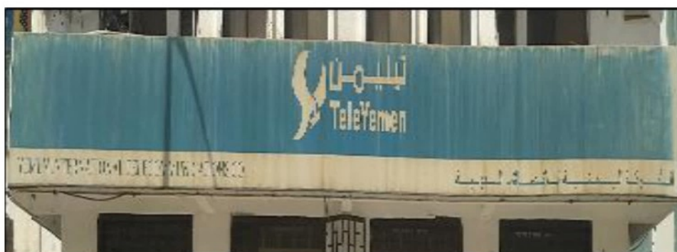
Figure 4.7 bilingual sign. Telecommunication centre sign.
